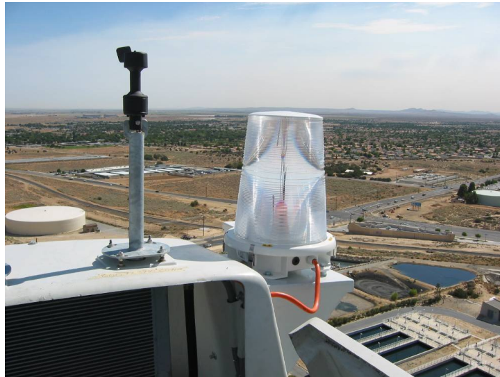
Figure 13b Typical Aviation Warning Light
