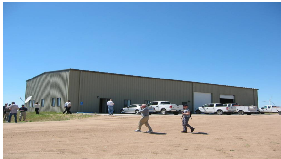
Figure 4c. Typical Operations and Maintenance Building
