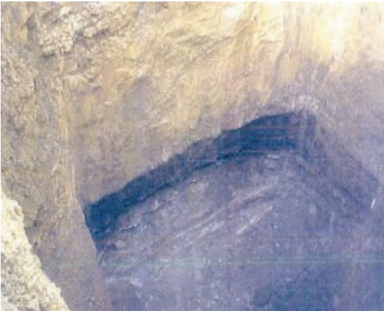
Figure 10. Excavation of Tower Foundation Hole Following Blasting
