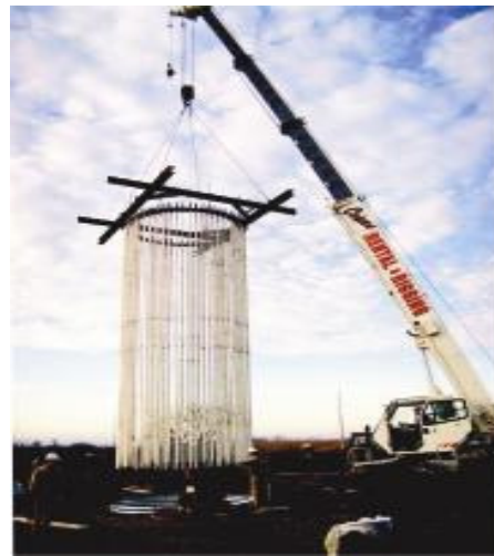
Figure 12. Bolt Structure for Tower Foundation
