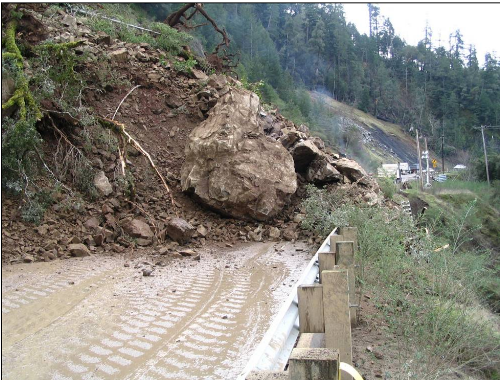
Figure 16-6: Confusion Hill Slide, view looking south on U.S. Highway 101, winter 2005-06.
