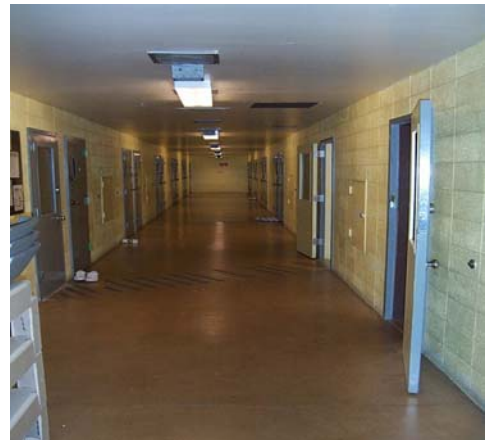
Juvenile Hall - after new lights installed
